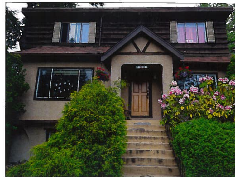
This house in the 3500-block West 35th Avenue in Vancouver is being torn down to be replaced by a bigger one. It sold for
